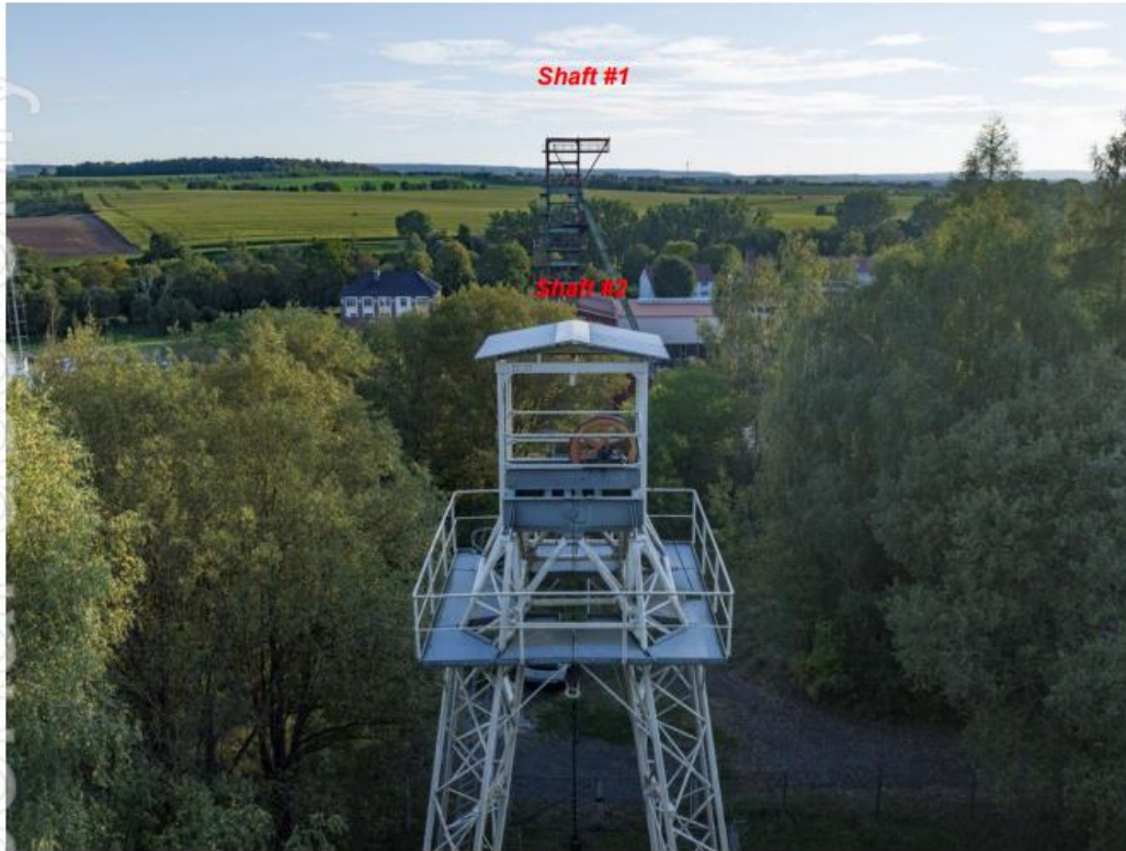
Image: Potential for existing shaft utilisation, South Harz Potash Ltd ASX Release February 2024
