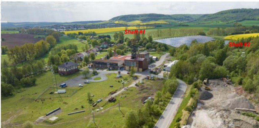
Image: Overview of surrounding infrastructure, South Harz Potash Ltd ASX Release February 2024
