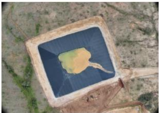
Figure 2: Brine dam commencing operation.
