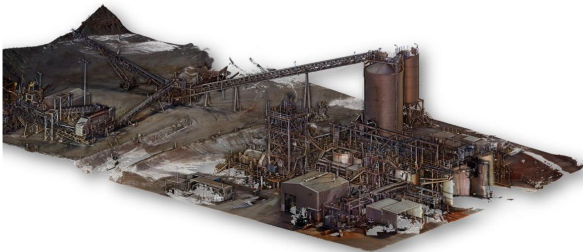
Image: 3D scan of Paulsen's processing facility as of February 2024, one of several assets owned by BlackCat Syndicate. March 2024 Paulsen's refurbishment update – ASX release.
