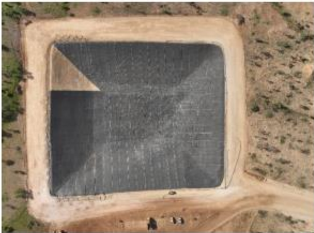
Figure 1: Brine dam nearing completion.
